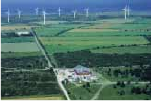
Figure 5. The Gotland VSC HVDC project in the foreground. Wind power in the background
