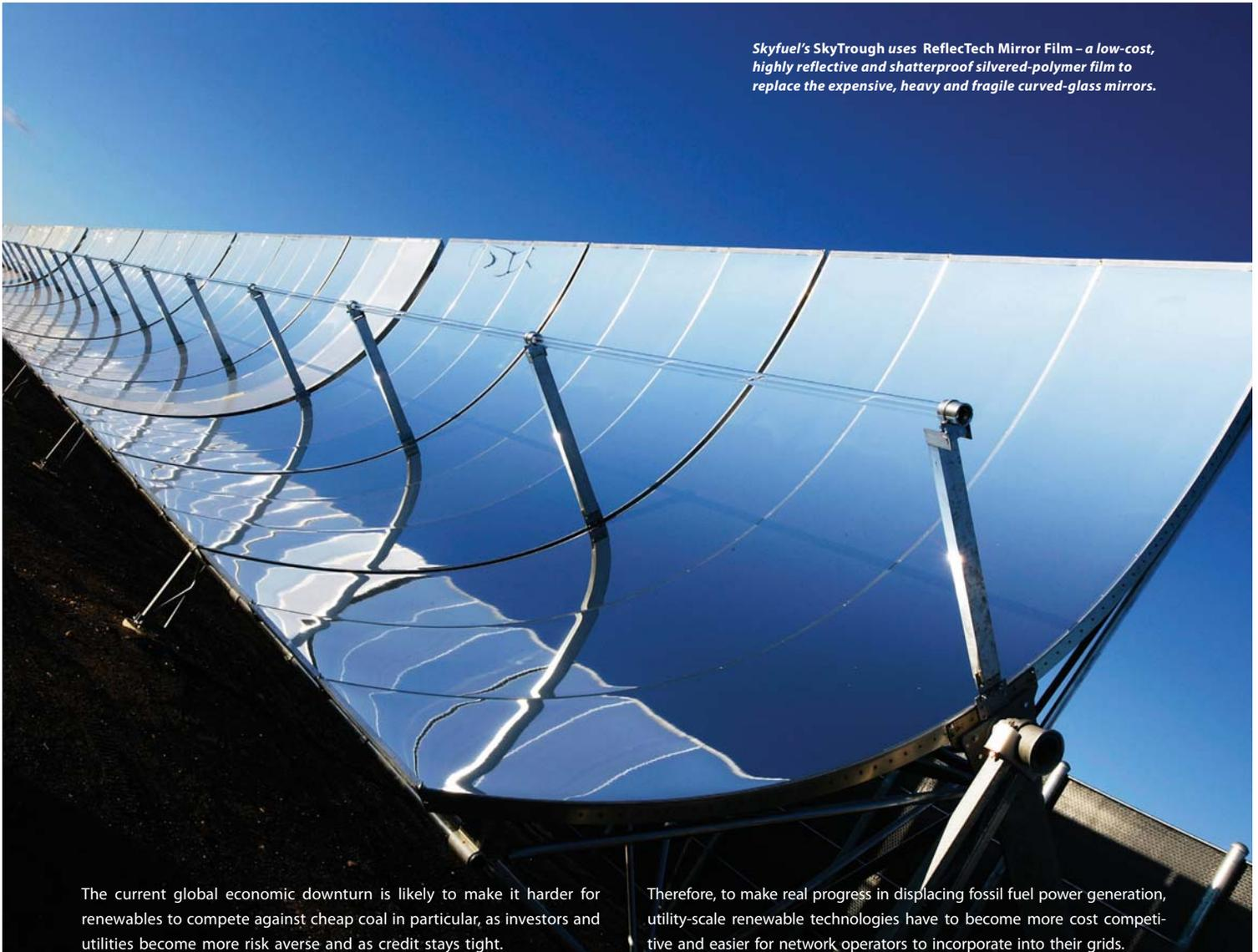
*Skyfuel's SkyTrough uses ReflecTech Mirror Film – a low-cost, highly reflective and shatterproof silvered-polymer film to replace the expensive, heavy and fragile curved-glass mirrors.*
