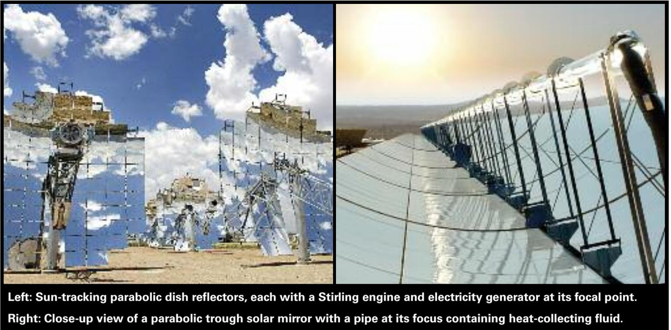
Left: Sun-tracking parabolic dish reflectors, each with a Stirling engine and electricity generator at its focal point.
